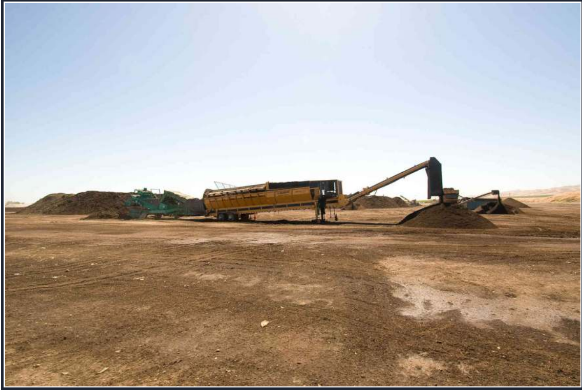
Figure 35: Central Valley Recology Facility Processing Compost Material
